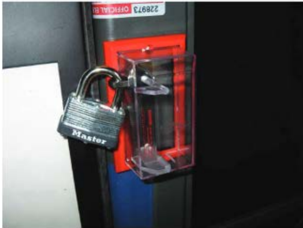
Figure 8.1 – Showing PEB slot covered with padlock type enclosure.
